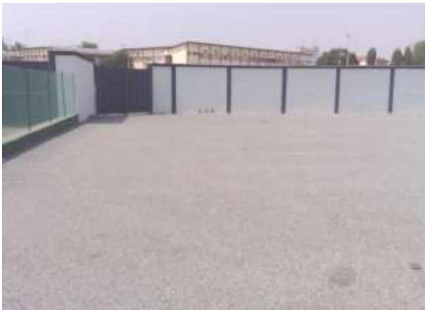
Figure. 1 Car Park covered with loose gravel (ASS) bays for PWDs (KSS)
