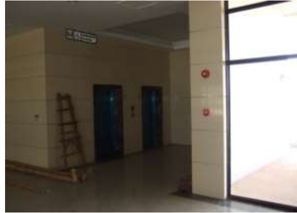
Figure. 14 Accessible lifts area with signage at TSS
