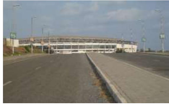
Figure. 4 Access route to STSS
