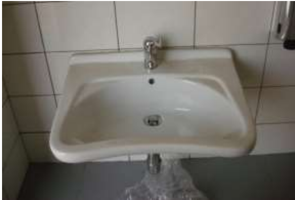
Figure. 19 Standard height wash hand basin handle for PWDs at KSS
